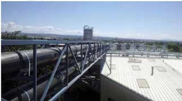
Cool Fit ABS Plus installed outdoors for the cooling unit of all the fermenting cellars at the Sierra Nevada Brewery.
